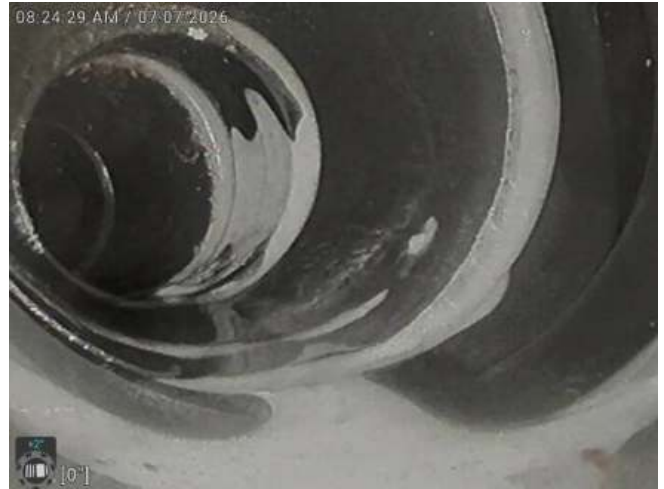
ABS PORTION OF BUILDING DRAIN CLEAN AND CLEAR IN GOOD STRUCTURAL CONDITION
