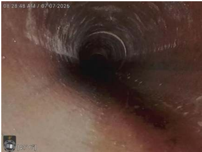
CLAY LATERAL PIPING CLEAN AND CLEAR
