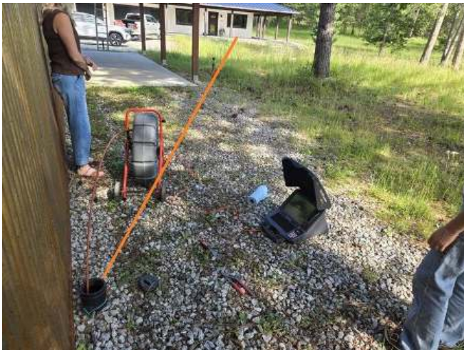
APPROXIMATE LOCATION OF SHOP LATERAL CLEANOUT LOCATION LOOKING NORTH TOWARD HOUSE
