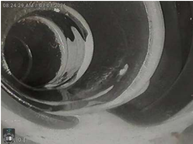
HOUSE LINE ABS PIPING - CLEAN AND CLEAR IN GOOD STRUCTURAL CONDITION
